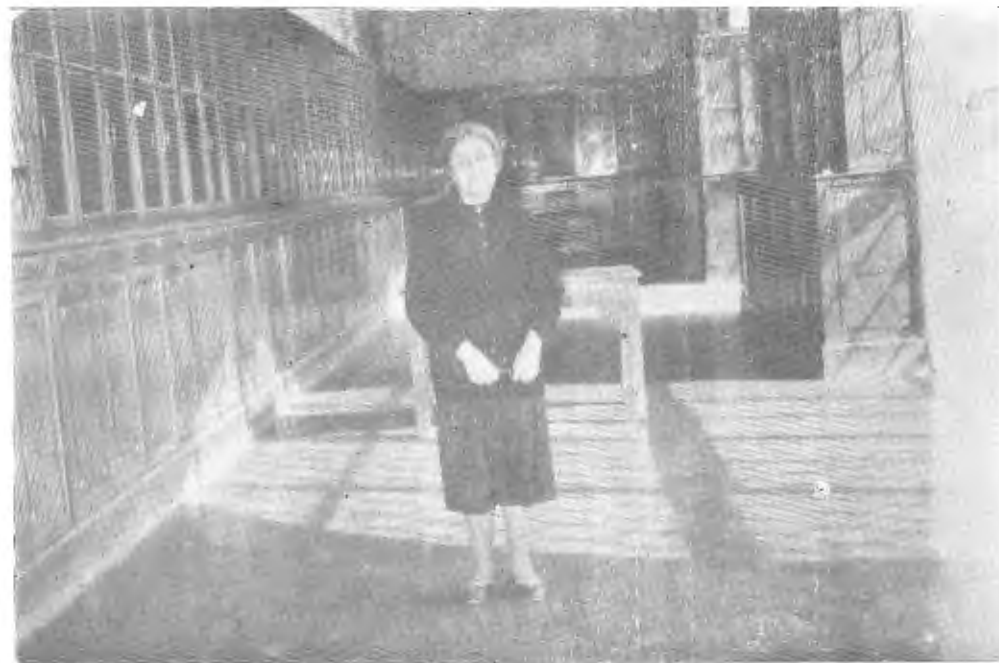
—The last inspection. —Northern side of the first floor bigger enlargement.
